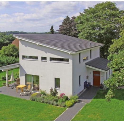
Hamdorf baut in Holztafelbauweise. Hamdorf builds in timber frame construction.
